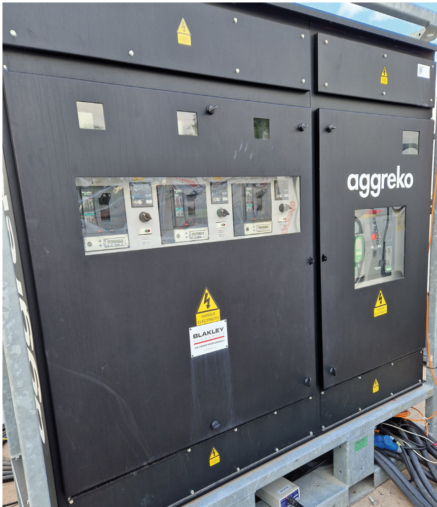
Figure 2 Rewireable metal-cased distribution unit
