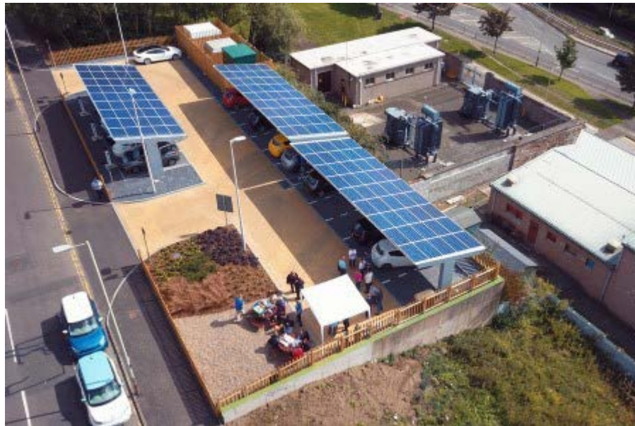
Figure 7.2 Dundee rapid charging hub case study. Reproduced by permission of Dundee City Council
