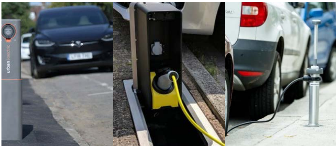
Figure 4.5 Low-impact infrastructure solutions: Urban Electric UEone , Streetplug and Trojan Energy . Reproduced by permission of Trojan Energy Limited
