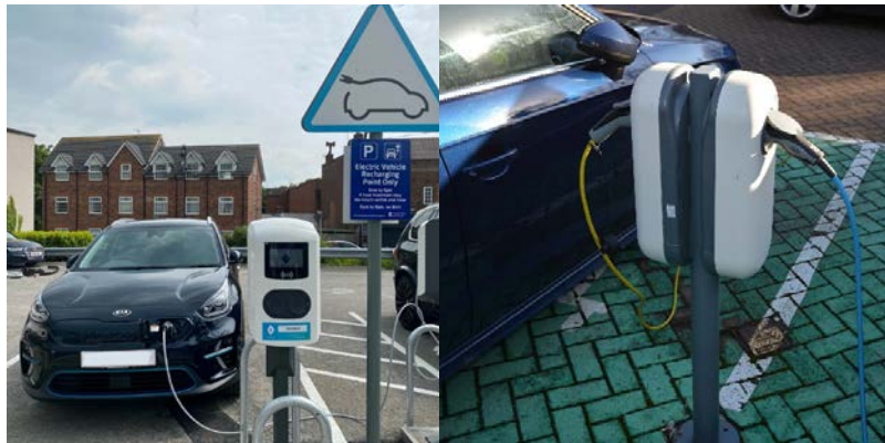
Figure 4.2 Example post/pedestal-mounted chargepoints
