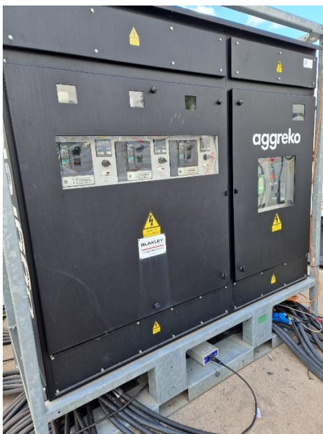
Figure 2 Rewireable metal-cased distribution unit
