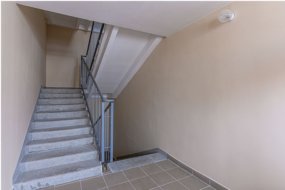
Figure 2: Protected escape stairs route
