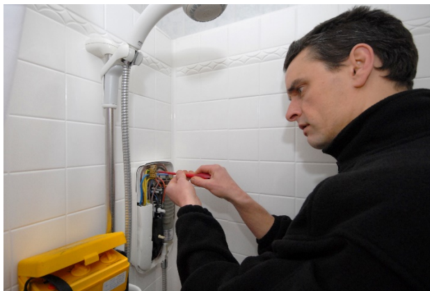
Fig 3 Consider how fixed electrical appliances forming part of the electrical installation are to be included, and if they have been subject to a manufacturer's safety recall
