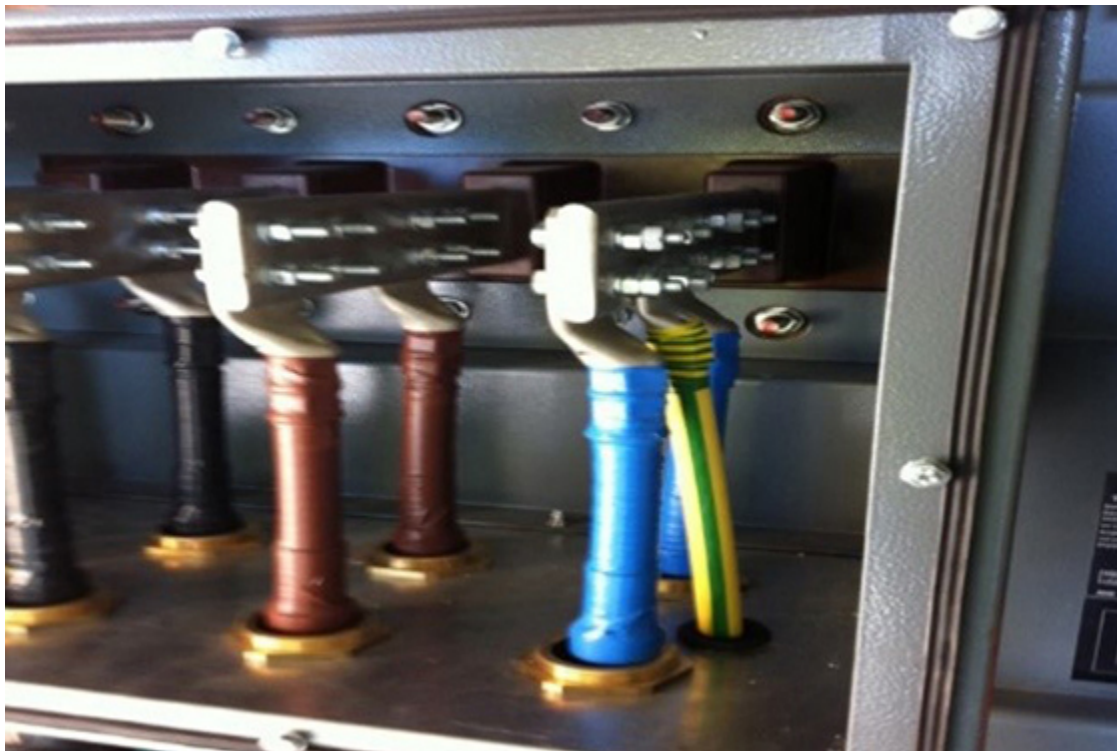
Figure 2: Transformer neutral to Earth connection inside transformer spill box
