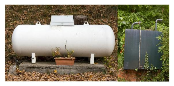
A separate earth rod is often seen installed at oil tanks but as the tank does not meet the definition of an extraneous-conductive-part, there is no requirement in BS 7671:2018 to provide protective bonding.
