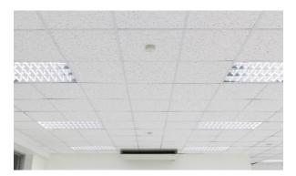
Similar to raised access floors, whilst suspended grid ceilings are metallic, they do not meet the definition of an extraneous-conductive-part. The luminaires will have circuit protective conductors installed but there is no requirement in BS 7671:2018 to install protective bonding to the ceiling grid.
