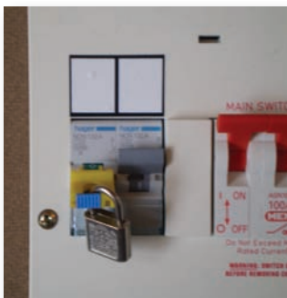
Examples of readily available lock-out devices for use with circuit-breakers
