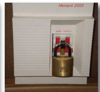
Universal lock-out device shown separately and securing a consumer unit main switch in the OFF position
