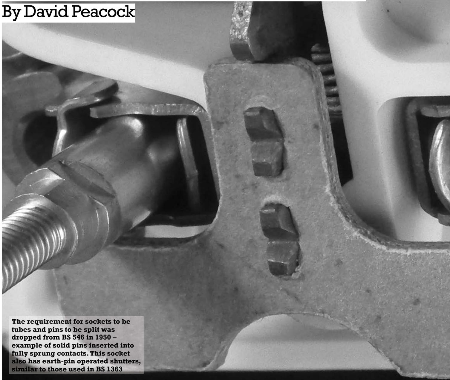
The requirement for sockets to be tubes and pins to be split was dropped from BS 546 in 1950 – example of solid pins inserted into fully sprung contacts. This socket also has earth-pin operated shutters, similar to those used in BS 1363
