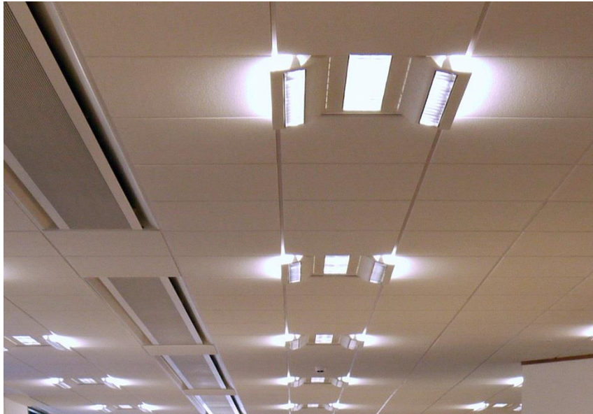
Image of lighting and mechanical services coordination
