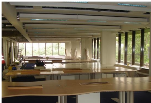
Image of integrated chilled beams being installed
