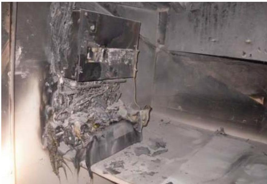
*This photo shows a fire involving a plastic consumer unit (bottom) and a metal consumer unit (top). In the experience of the LFB, when a fire originates within a metal consumer unit (even without sealed grommet holes and the plastic MCB cover failing), the fire is still generally contained to the consumer unit.*
