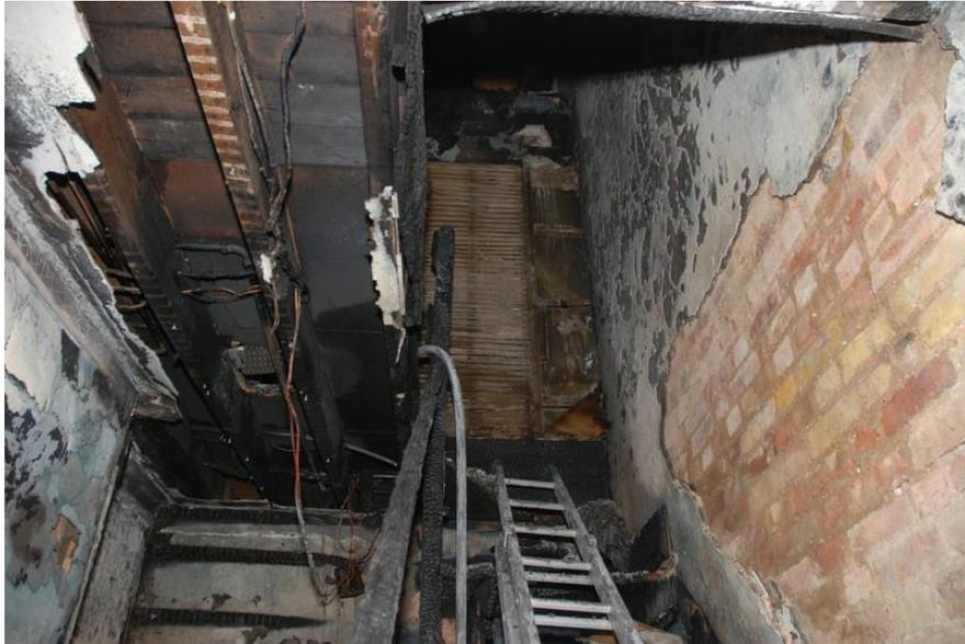
*Following a fire under the stairs, the stair treads have burnt through, the ceiling has failed and the plaster has come off the wall.*
