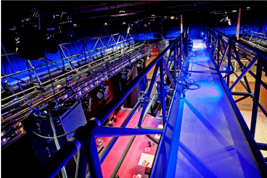
Lighting bridges above the auditorium at Mareel Arts Center, Lerwick ©Phatsheep
