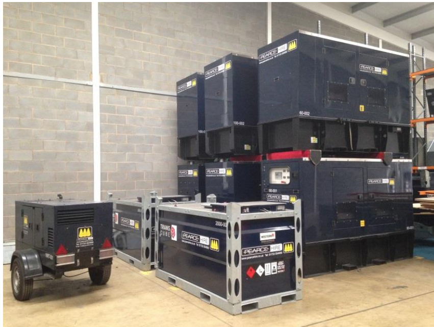
Pearce Hire warehouse - generators and fuel tanks ready for hire!
