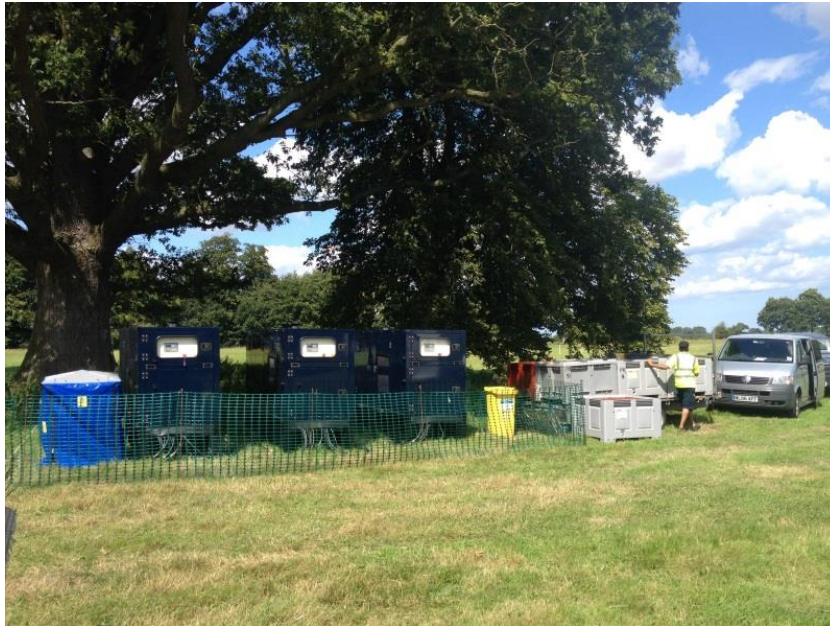
Blickling Hall Proms concert - three generators in synchronised set up
