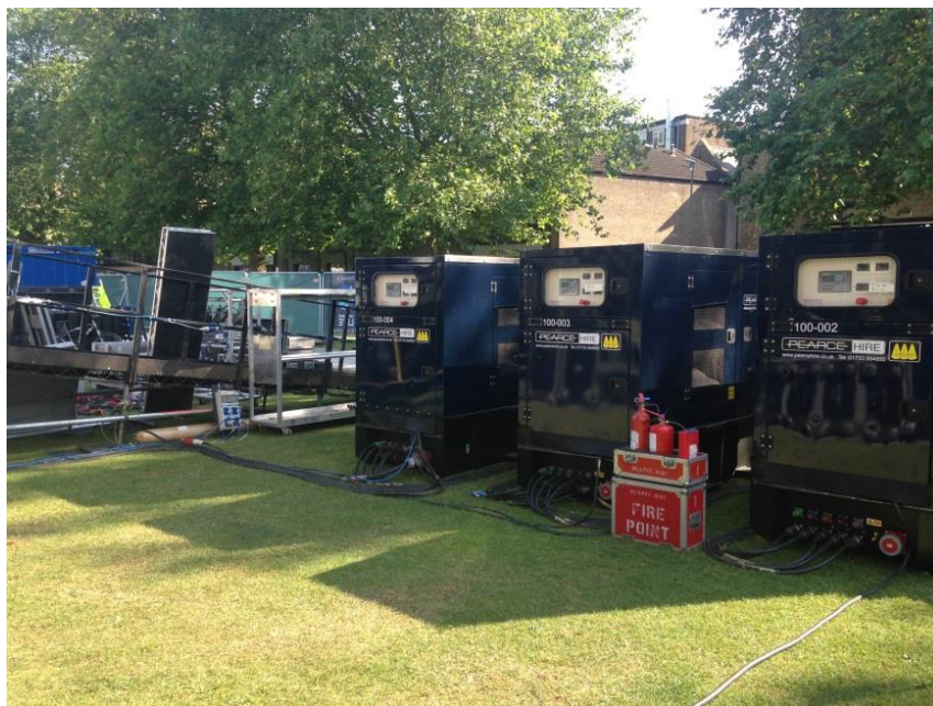
Pop in the Park Cambridge - triple synchronised generator set up
