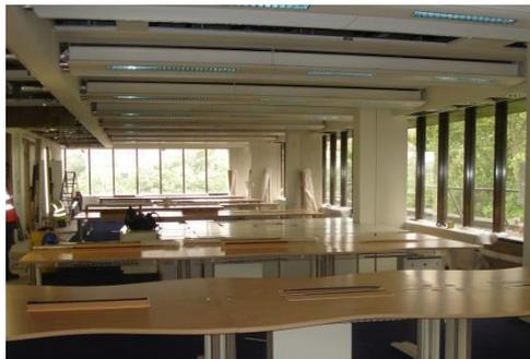
*Image of integrated chilled beams being installed*
