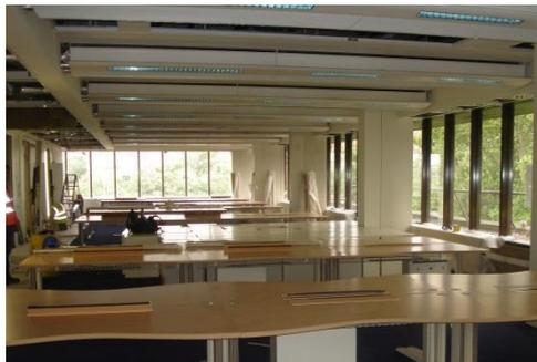
*Image of integrated chilled beams being installed*
