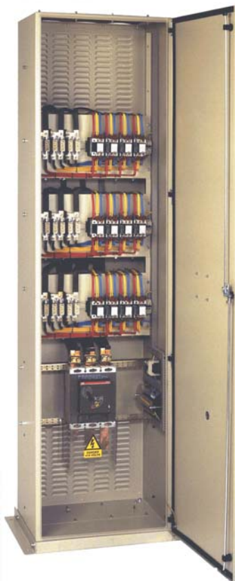
A 324 kVAr, automatic power factor correction unit.
