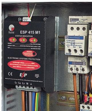
**Installation of a surge protective device**
