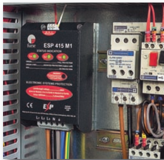
Installation of a surge protective device
