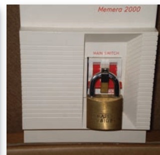
Universal lock-out device shown separately and securing a consumer unit main switch in the OFF position
