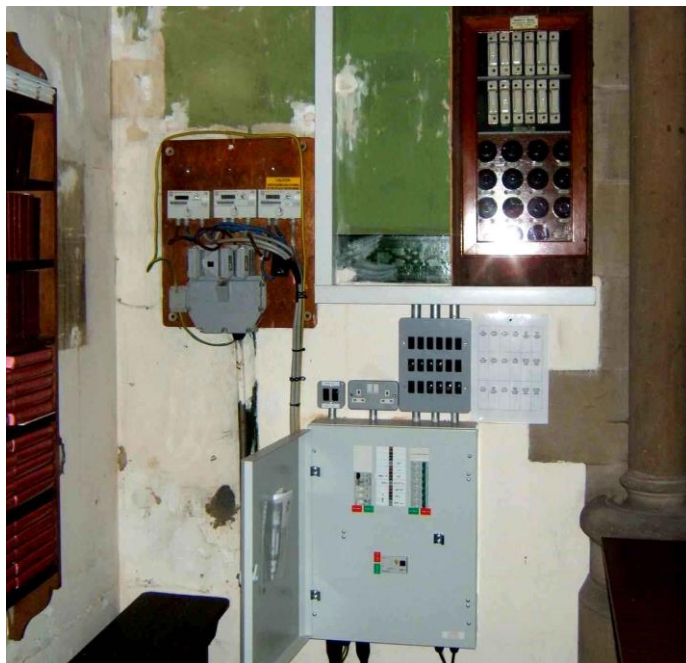
Grosmont St Matthew after rewiring. Picture courtesy of D Haddon-Reece.
