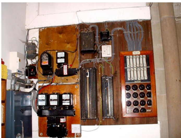
Grosmont St Matthew before rewiring. Picture courtesy of D Haddon-Reece.
