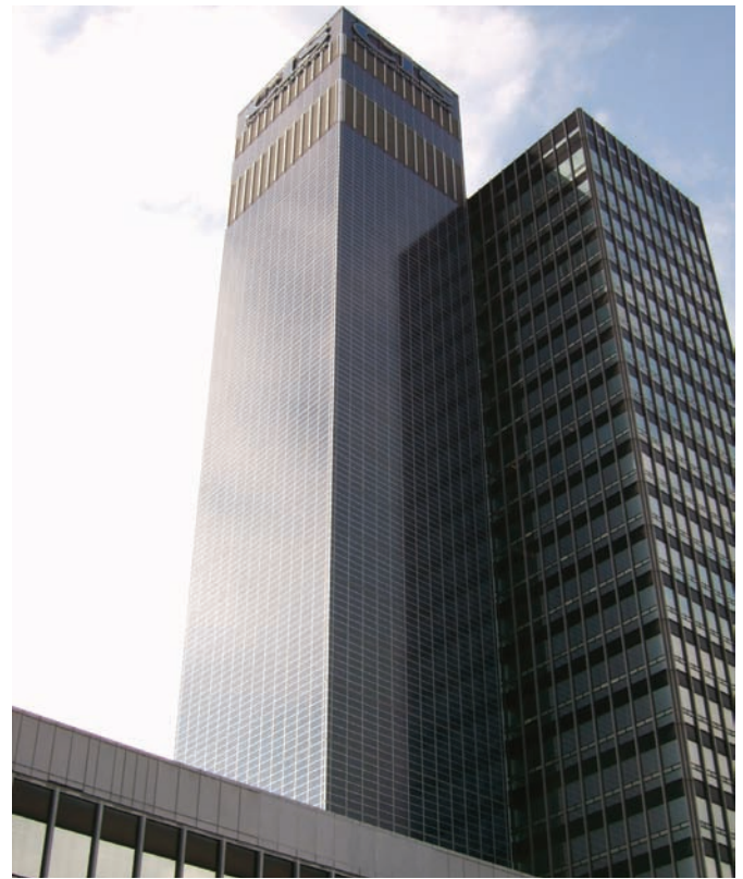
PV system incorporated into a building
