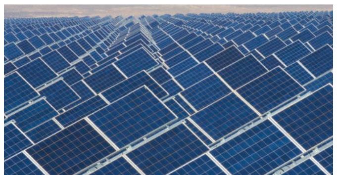
Large array installation
