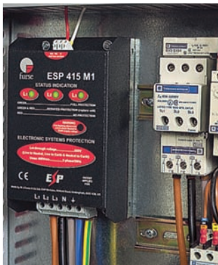
Installation of a surge protective device
